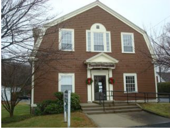
FAYVILLE VILLAGE HALL
