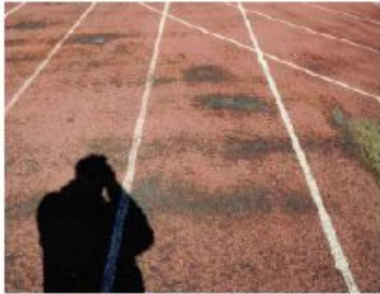
WEAR ON TRACK SURFACE
