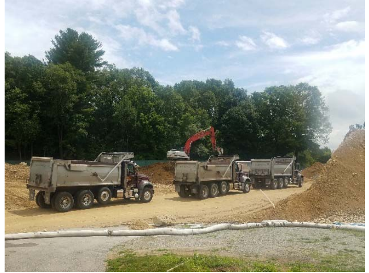
Photo depicts the removal of excess loam from the site on 7/25/28.
