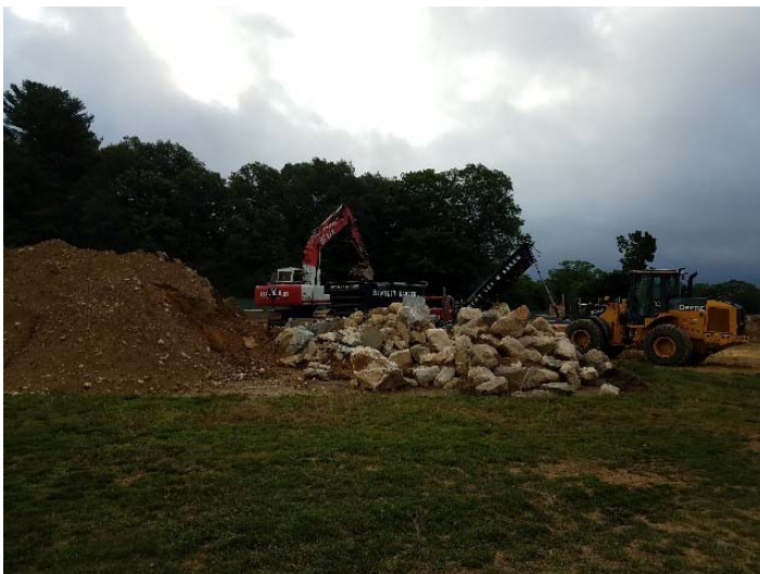
Photo depicts the excavated site rocks and boulders on 7/26/18.
