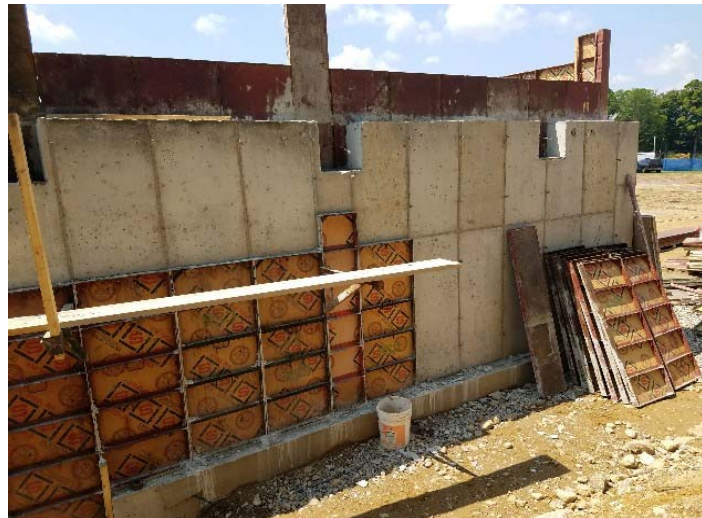
Picture: Relocated Golf Clubhouse foundation walls.
