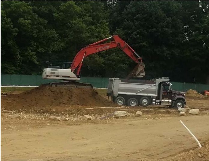
Photo depicts the loading of excess loam from the site on 7/26/18.
