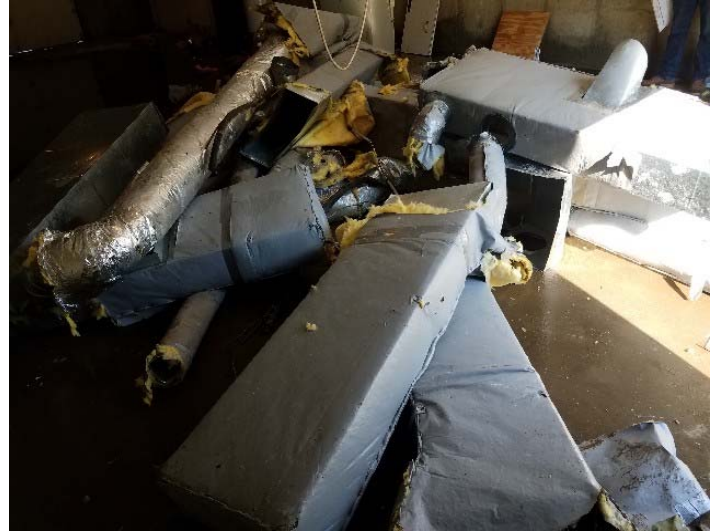
Photo depicts the demo Golf Clubhouse AC ducts on 7/27/18..
