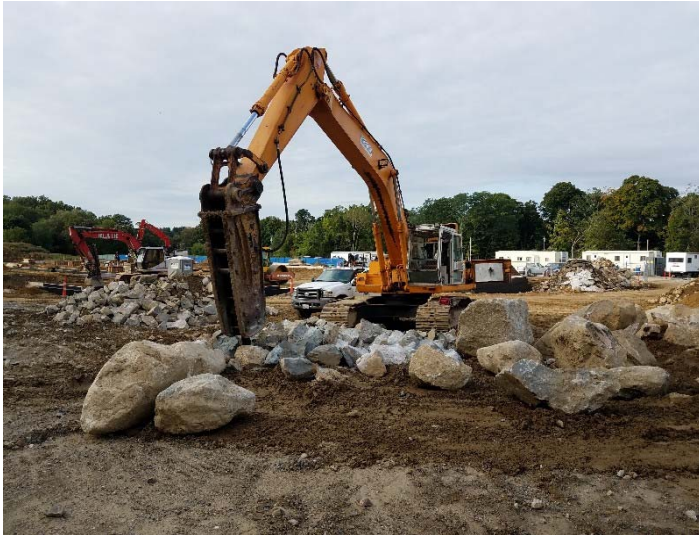
Photo depicts the breaking of large boulders on 9/21/18.
