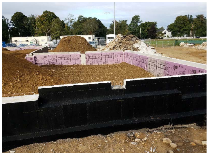
Photo depicts the backfill foundation wall on 9/21/18.
