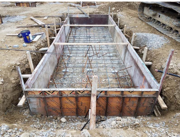
Photo depicts large interior footing rebar on 9/24/18.
