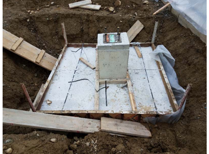
Photo depicts the interior footing construction on 9/26/18..
