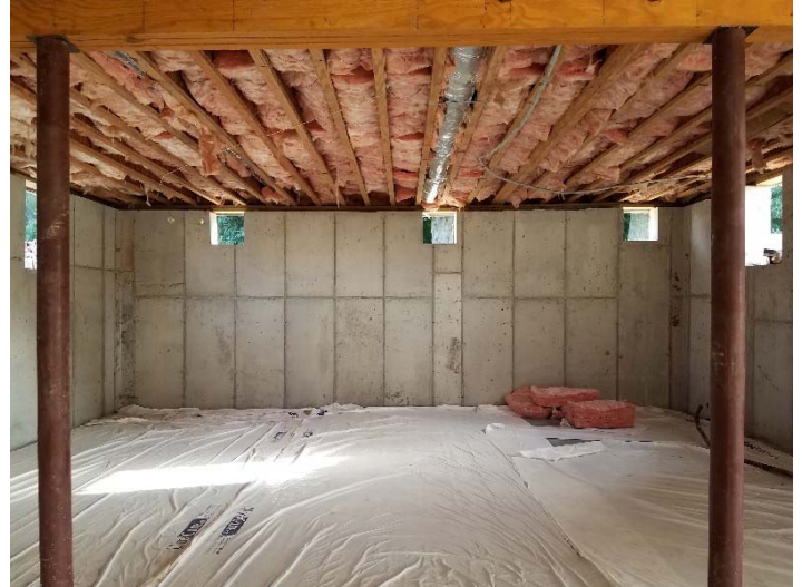
Photo depicts the Golf Clubhouse basement concrete on 9/06/18.
