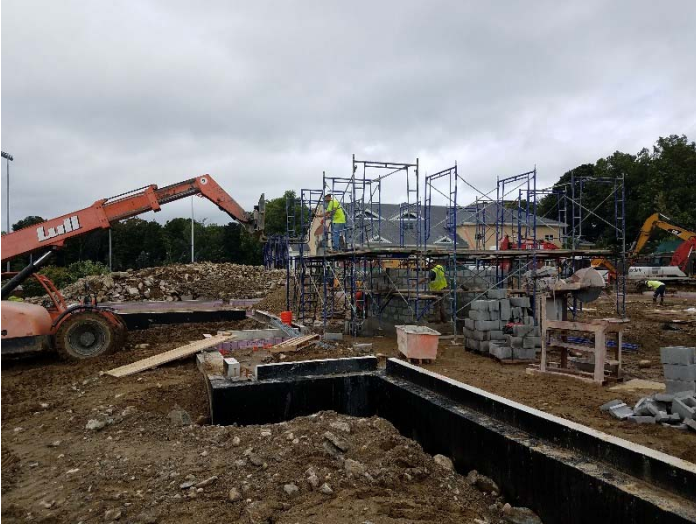
Photo depicts elevator shaft cmu erection on 9/26/18.
