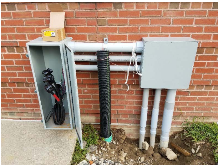
Photo depicts Woodward School septic conduits rough-in on 9/21/18.
