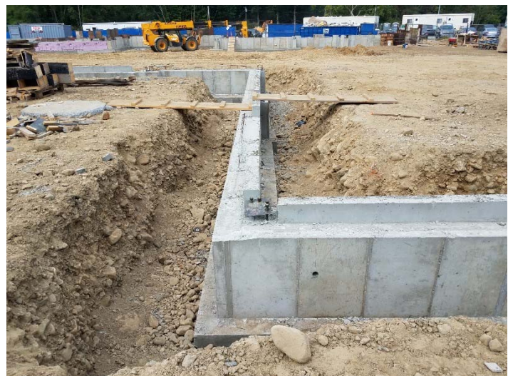
Photo depicts the foundation stem wall on 9/05/18.
