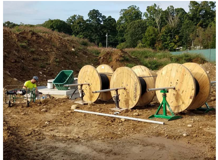
Photo depicts pulling of the septic wiring on 9/22/18.
