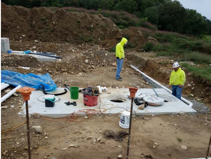
Photo depicts the septic tank filling on 9/24/18.
