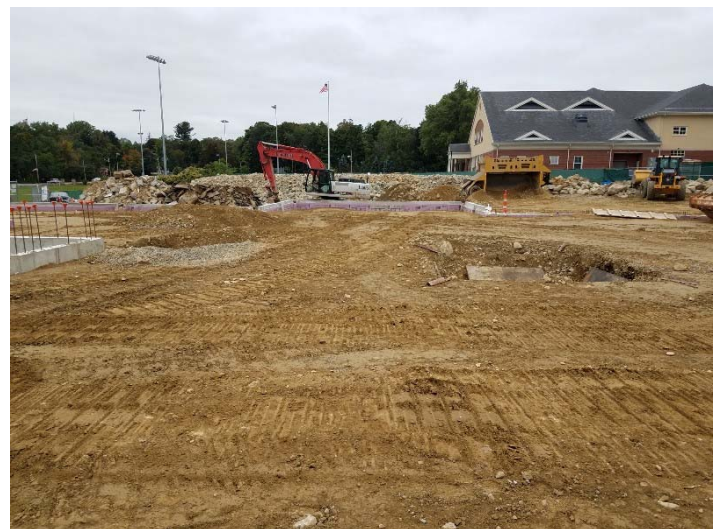
Photo depicts the interior foundation footings on 9/24/18.
