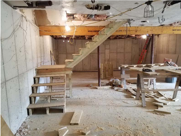
Photo depicts the Golf Clubhouse interior stair on 9/20/18.
