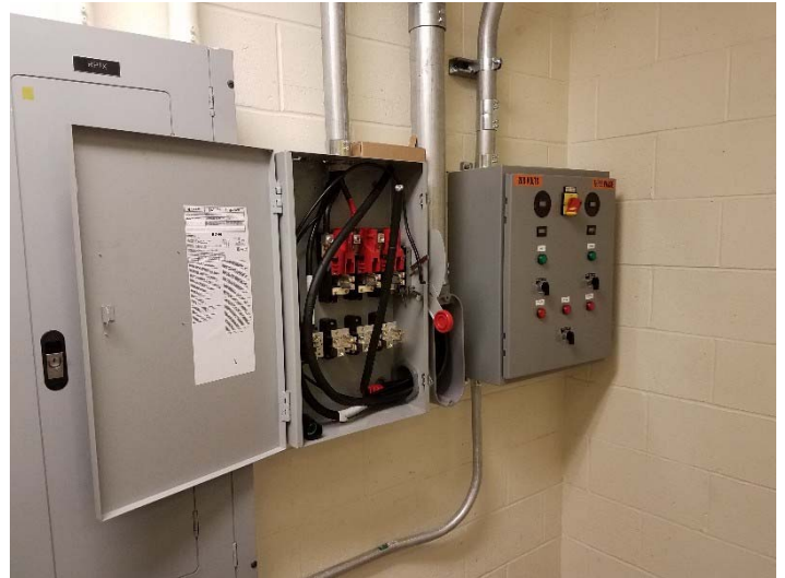
Photo depicts the septic monitoring panel on 9/19/18.
