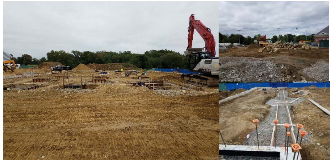
Pictures: Interior foundation footings, ledge and boulders, forming foundation footings.
