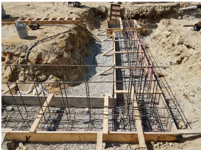
Photo depicts the foundation wall footings on 9/04/18.
