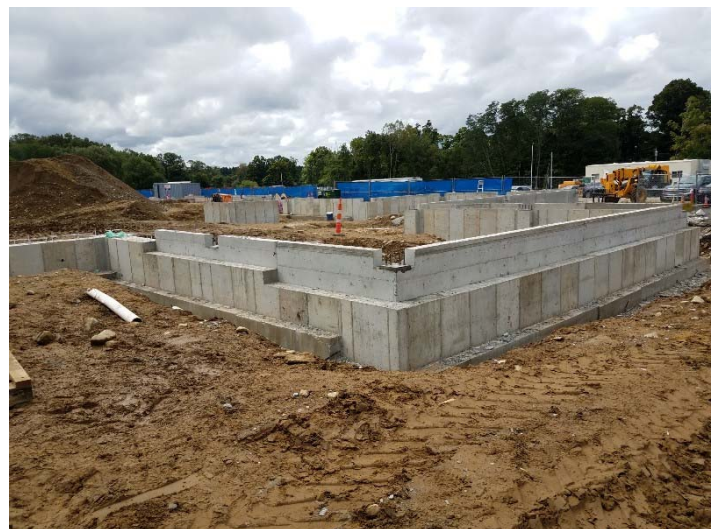
Photo depicts the foundation walls on 9/14/18.
