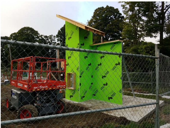
Photo depicts the Mockup Location on 9/17/18.
