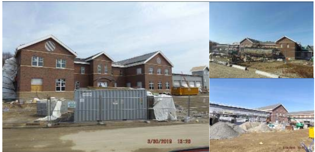
Pictures: Overall building progress
