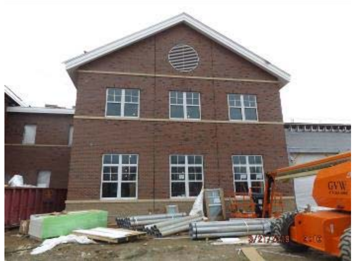
Photo depicts the installation of windows.
