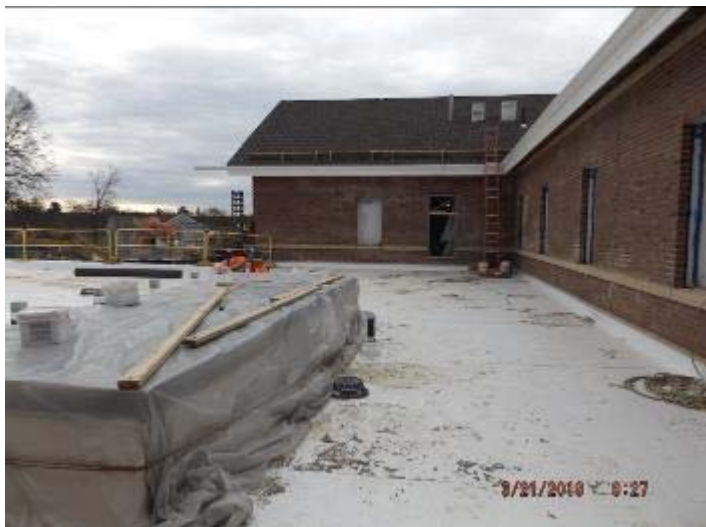
Photo depicts the progress of the lower flat roof.
