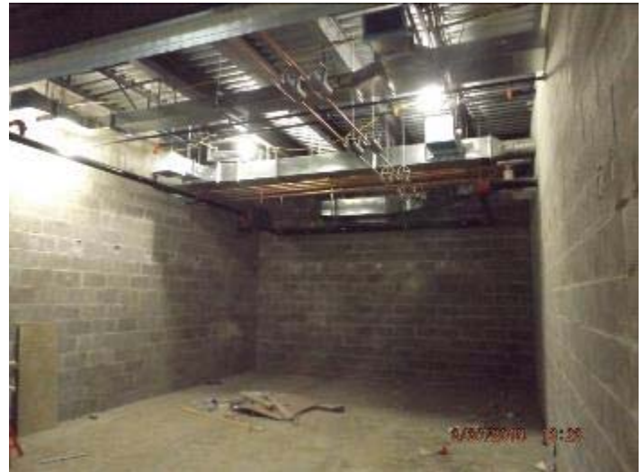
Photo depicts the progress of first floor turnout gear room.
