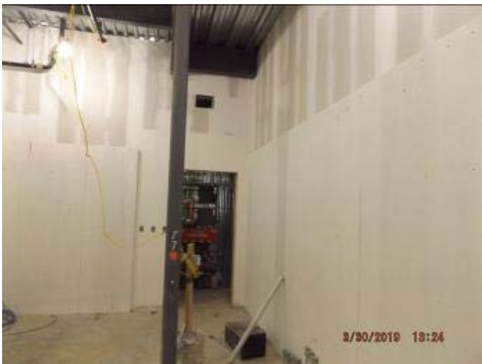
Photo depicts the progress of the first floor electrical room
