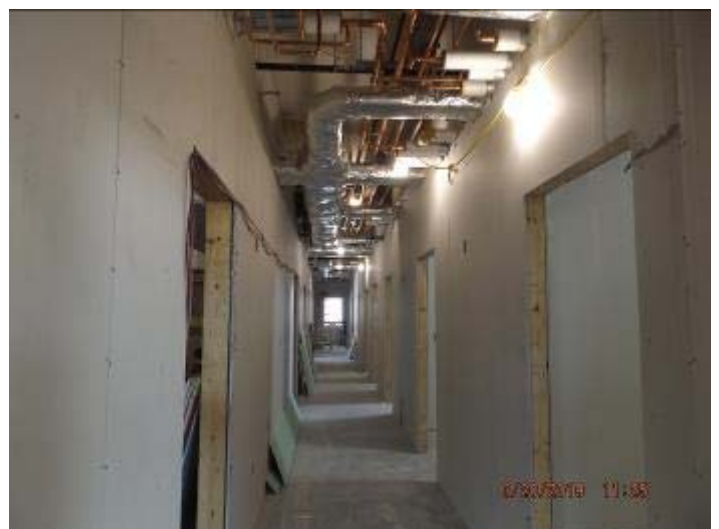
Photo depicts the progress of the second floor dorm room hallway
