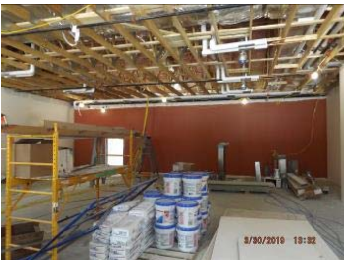
Photo depicts the progress of second floor fitness room.
