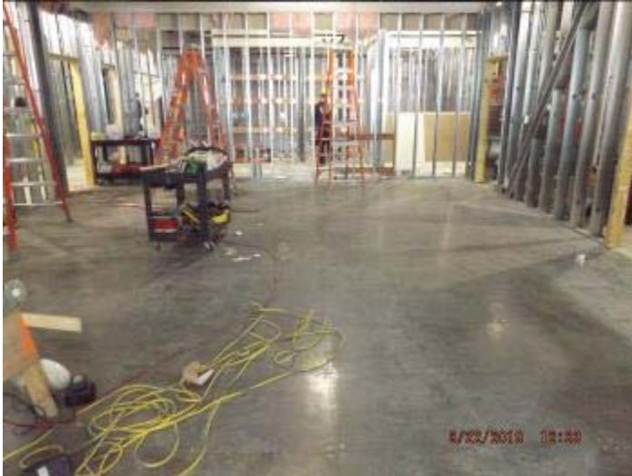
Photo depicts the progress of first floor dispatch area.
