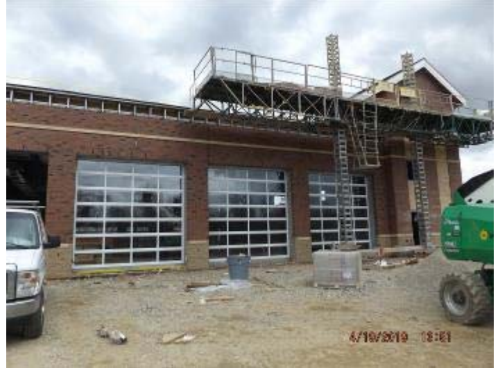
Photo depicts the installation of the garage doors
