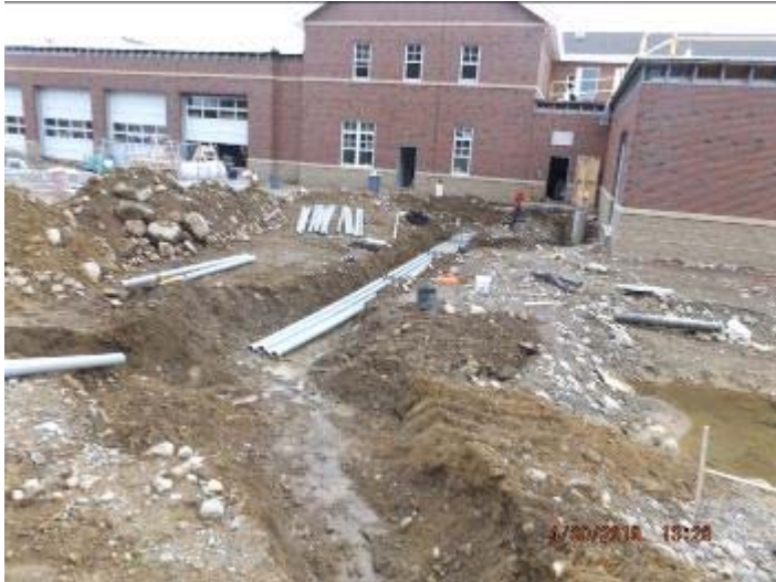
Photo depicts the progress of excavation for generator pad
