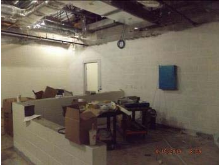
Photo depicts the progress of the booking area
