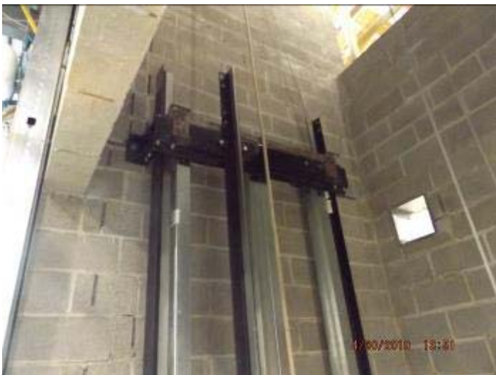
Photo depicts the progress of the elevator.
