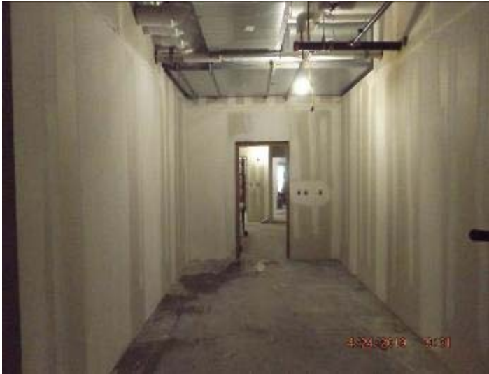
Photo depicts the progress of the first floor.
