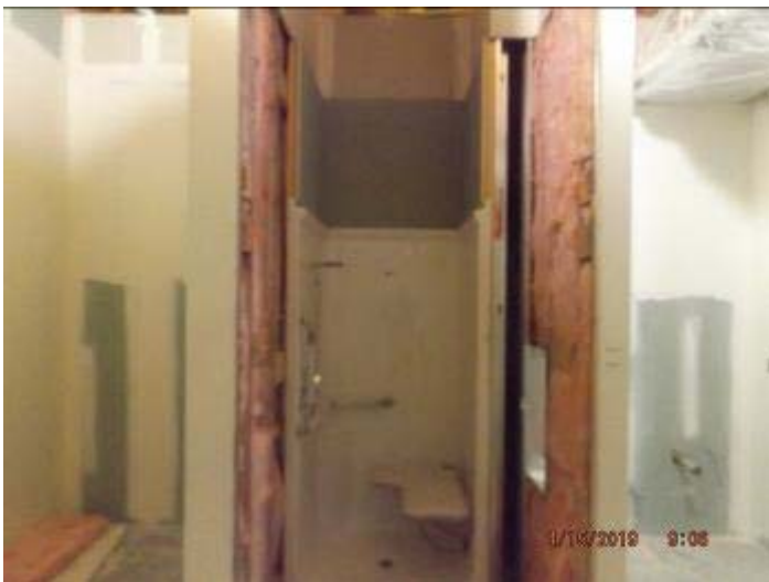
Photo depicts the progress of plumbing fixtures on the second floor
