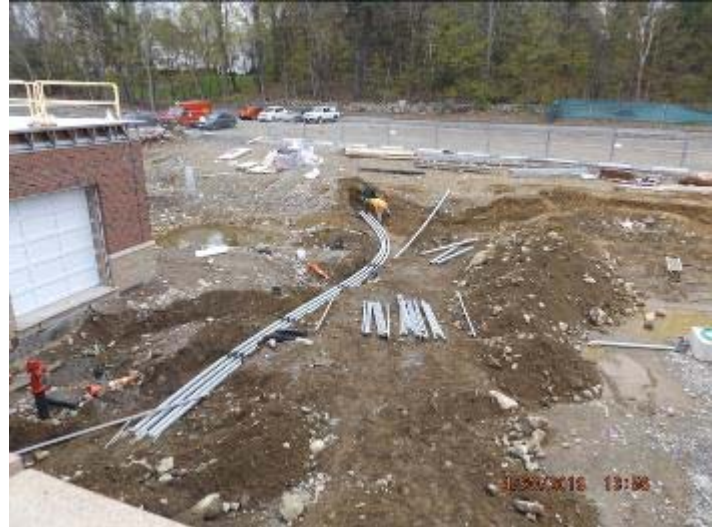
Photo depicts the progress of excavation, and conduit installation.
