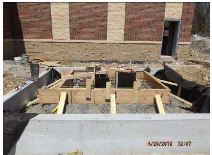
Photo depicts transformer pad prep.
