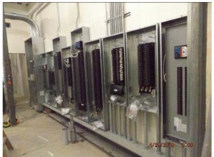
Photo depicts the progress of the electrical room.
