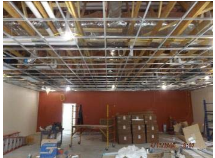
Photo depicts the progress of the fitness room
