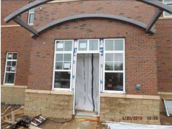
Photo depicts the progress of the exterior at the main entrance.
