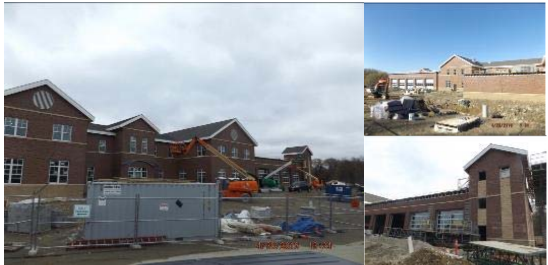
Pictures: Overall building progress
