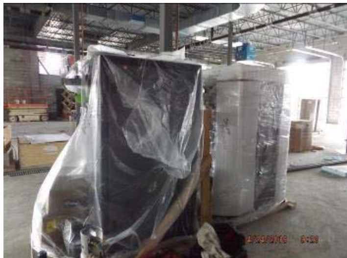
Photo depicts the delivery of main mechanical room equipment
