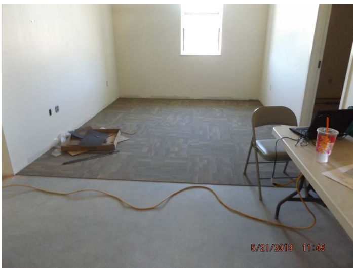
Photo depicts the progress of the second floor carpet.
