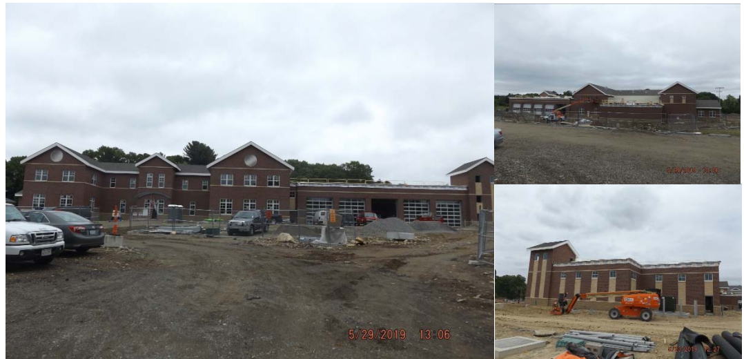
Pictures: Overall building progress
