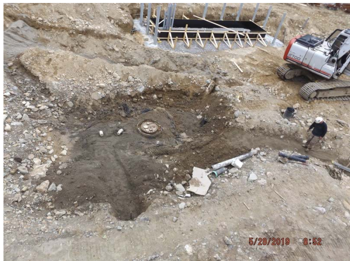
Photo depicts the progress of the generator pad, and tight tank.
