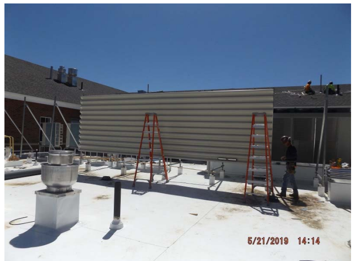
Photo depicts roof screen, and antenna bracket installation.
