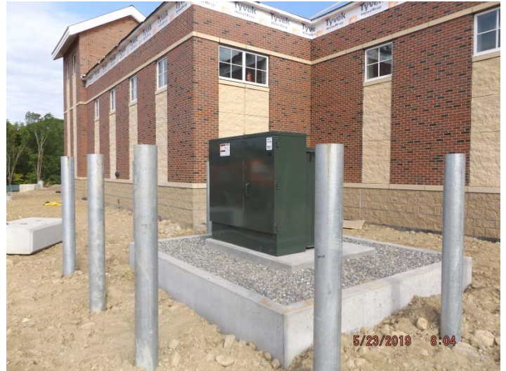
Photo depicts the installation of the transformer.
