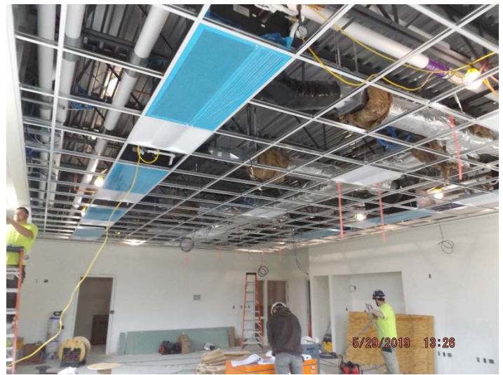
Photo depicts the progress of the training room.
