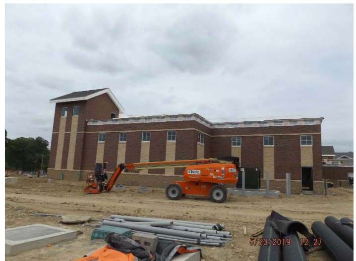
Photo depicts exterior progress on the east side of the building.
