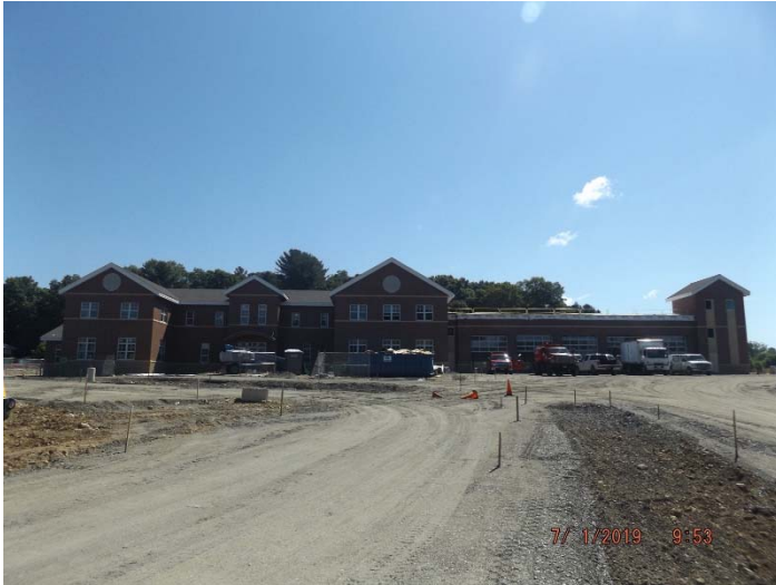
Photo depicts the progress of the exterior of the front of the building.
