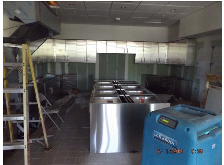
Photo depicts the progress of the kitchen
