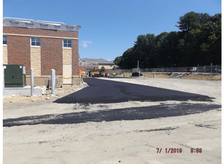
Photo depicts the progress of asphalt
