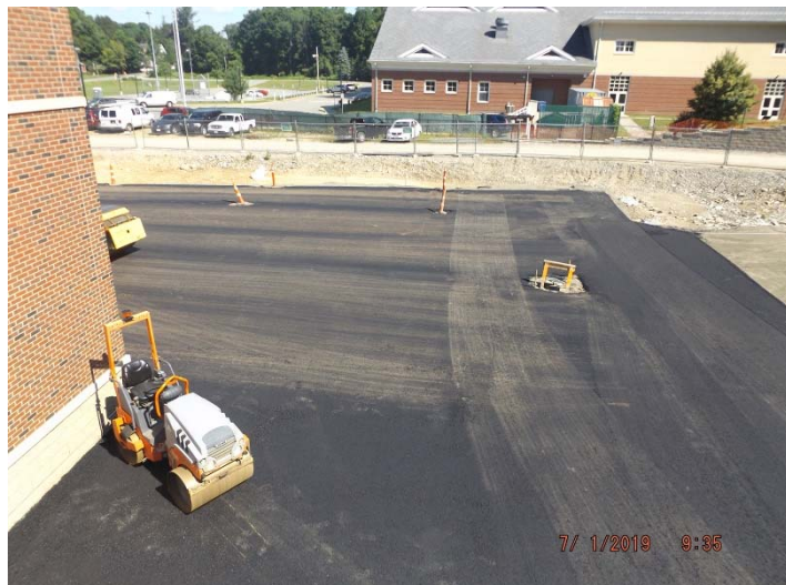
Photo depicts the progress of asphalt, and footings ready for carport steel
