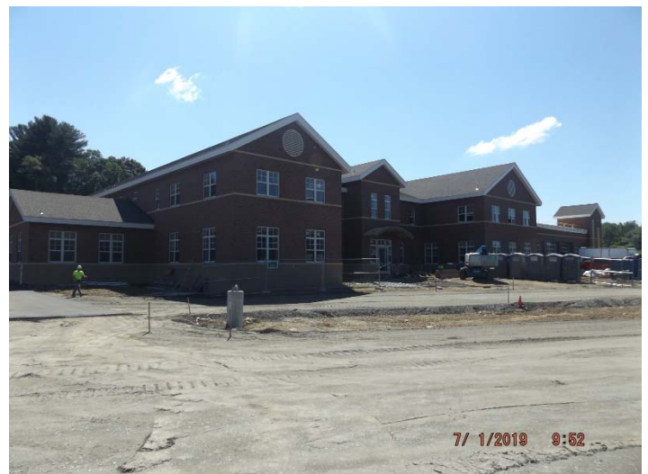
Photo depicts exterior progress around main entrance
