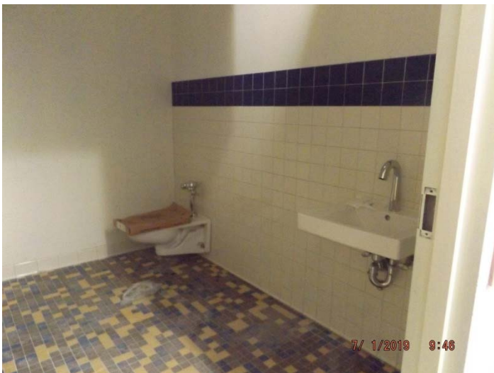
Photo depicts the progress of restrooms throughout building
