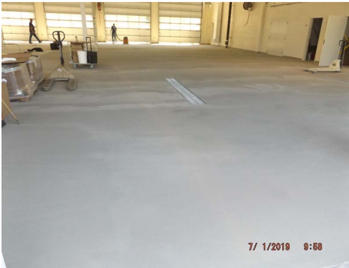
Photo depicts the progress of the apparatus bay floor
