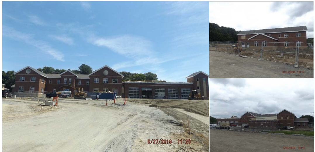
Pictures: Overall building progress
