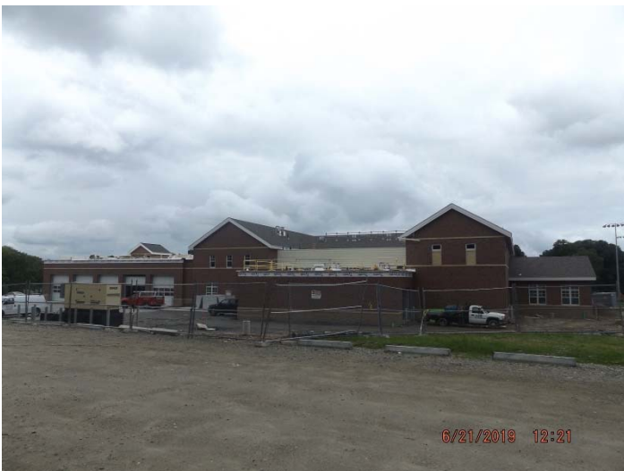
Photo depicts the progress of the exterior of the rear of the building.
