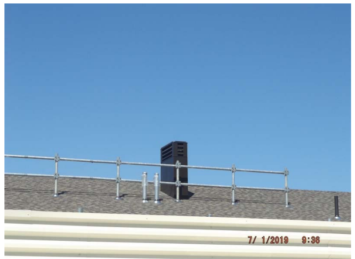
Photo depicts the completion of the elevator damper.
