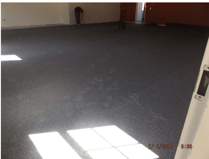
Photo depicts the progress of the fitness room floor
