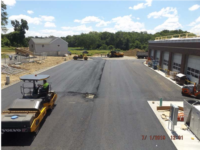
Photo depicts the progress of asphalt
