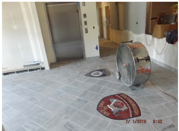
Photo depicts the progress of the lobby floor.
