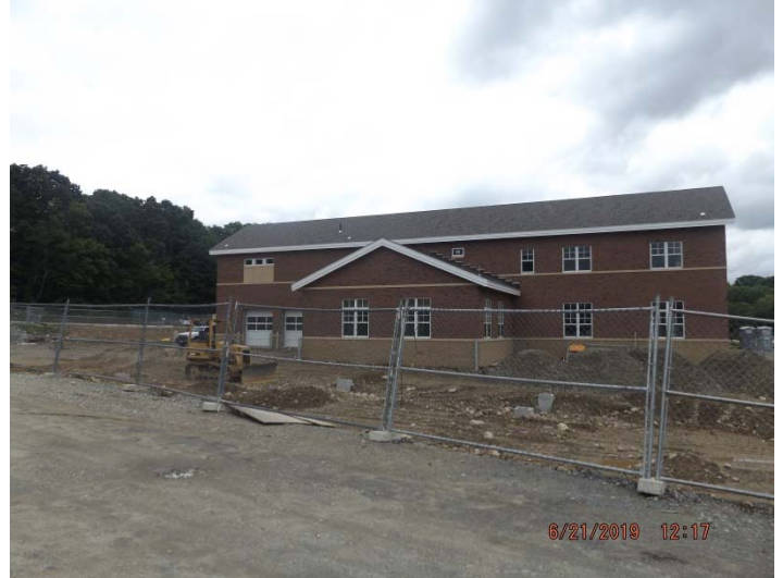
Photo depicts the exterior progress on the west end of the building.
