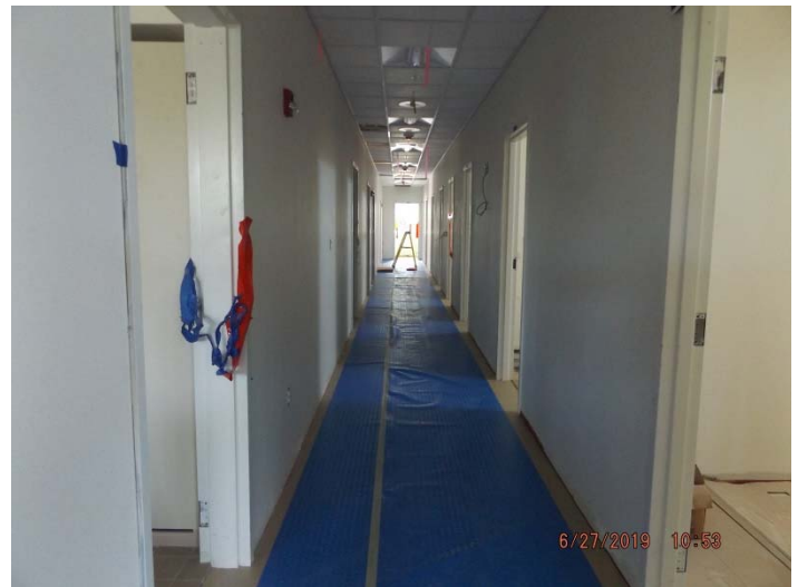
Photo depicts the finished/protected flooring on the second floor.
