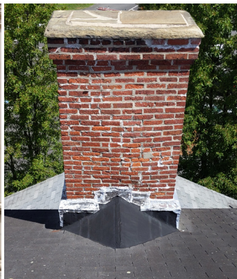
Deteriorated chimney flashing and roofing have reached the end of their lifespan.
