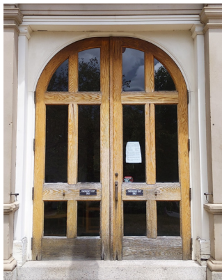
Exposed wood doors are left worn and severely water-damaged.
