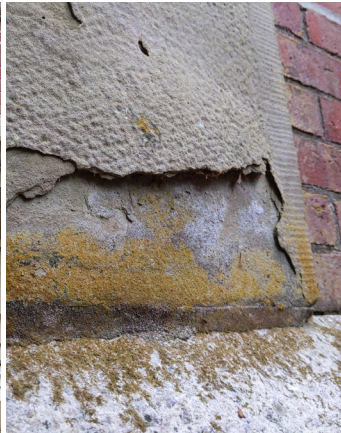
Rainwater-soaked sandstone blocks are spalled and cracked due to leaking downspouts.
