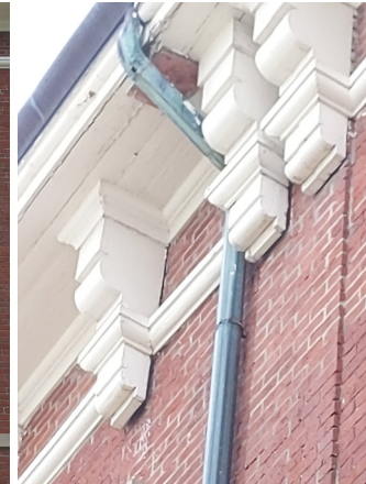
Woodwork at the building cornice shows signs of damage. Paint is worn and chipped.
