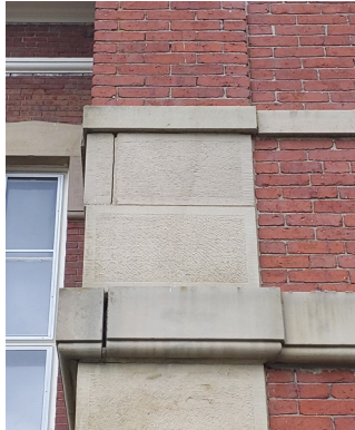
Sandstone mortar joints are open and at risk for water infiltration.
