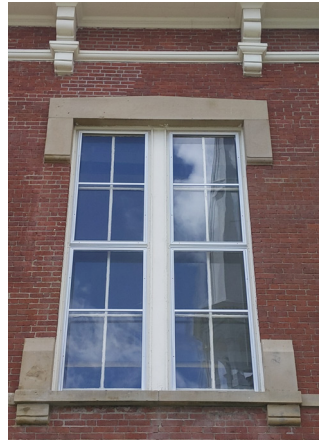
Monolithic windows are deteriorated, energy inefficient, and inoperable. Exact replicas of the originals, properly aligned for easy operation will be produced.
