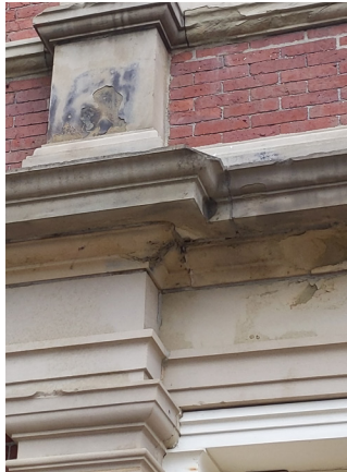
Sandstone trim is eroded and damaged from years of rainwater washing across its face.
