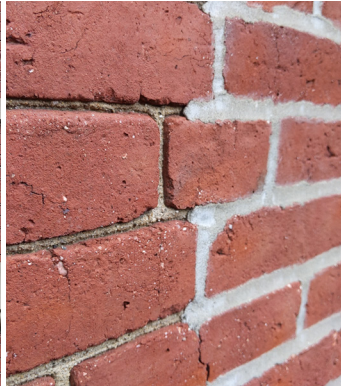
Brick mortar is deteriorated or repointed with incorrect color in hard mortar.
