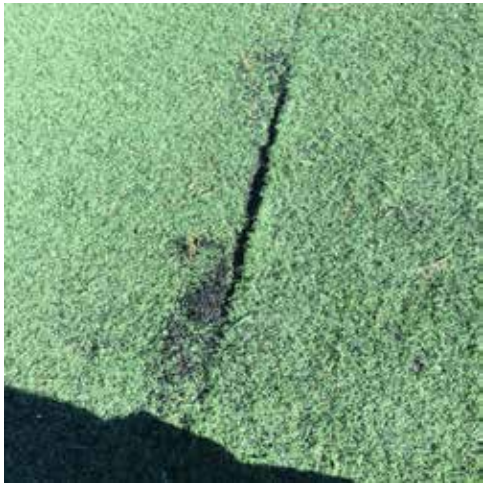
TEAR IN TURF FABRIC
