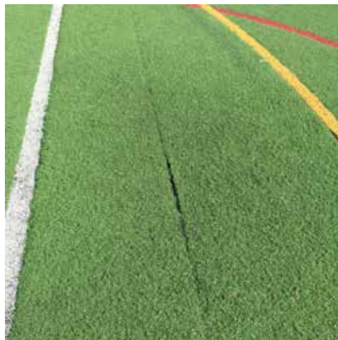
TEAR IN TURF FABRIC
