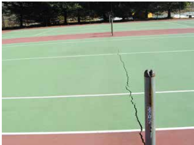
CRACKING AT TENNIS COURTS
