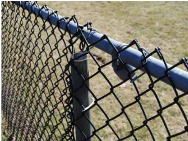
DISCONNECTED FENCE
