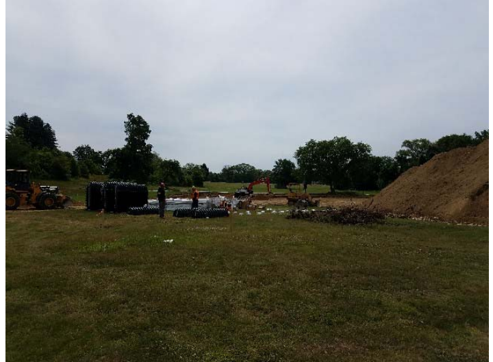
Photo depicts the septic field excavation work and septic chambers, piping, accessories.
