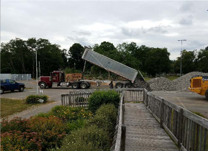
Photo depicts the delivery of the double washed crushed stone on 6/25/18.
