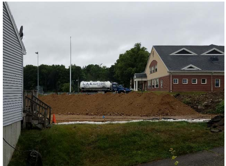
Photo depicts the sewage tanks pumping of Woodward School on 6/28/18.
