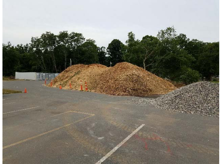
Photo depicts the tree cutting chipping mulch pile prior to hauling off the site on 6/26/18.
