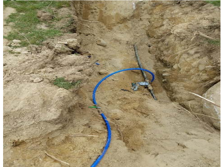
Photo depicts the tracing and connection of the Golf Clubhouse waterline on 6/25/18.
