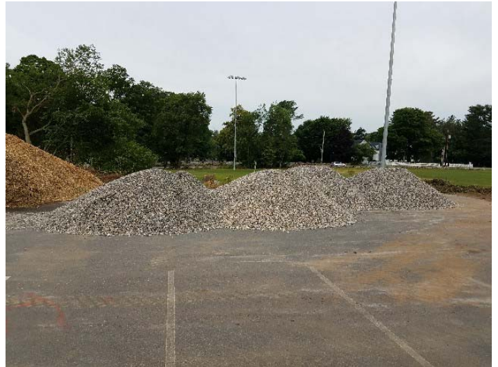
Photo depicts the delivered double washed crushed stone for the septic field chamber base course on 6/26/18.
