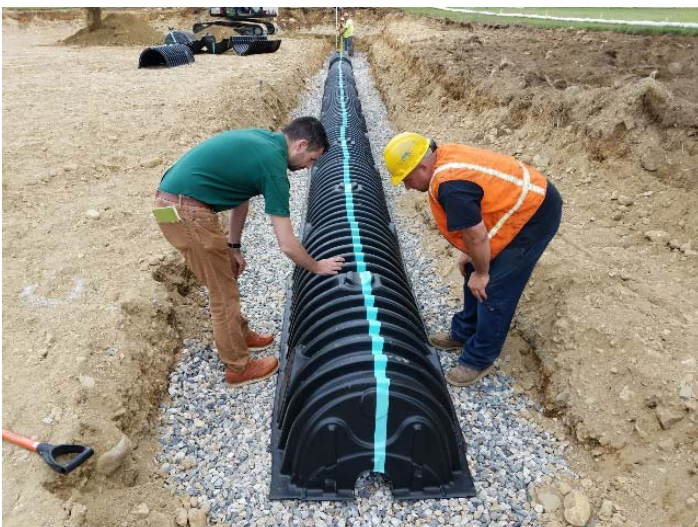
Photo depicts the septic field installation of the septic chambers for civil engineer inspection on 6/27/18.
