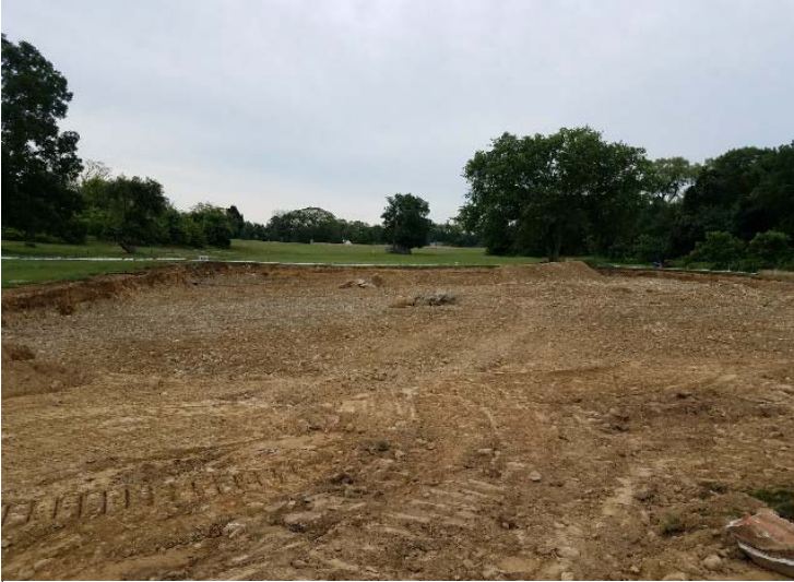
Photo depicts the septic field excavation, prior to trench excavation for the septic chambers on 6/26/18.
