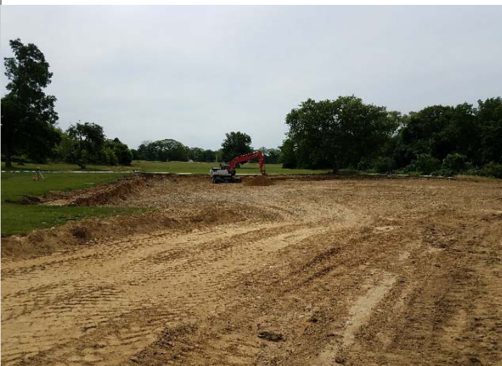
Photo depicts the septic field trenching for the septic chambers on 6/27/18.
