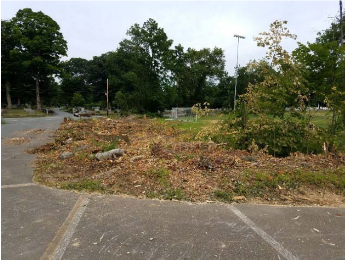
Photo depicts the tree cutting and clearing adjacent to the Woodward School soccer field on 6/25/18.
