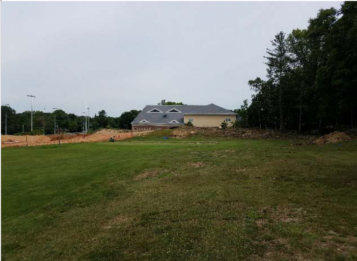
Photo depicts progress of the tree cutting work adjacent to Woodward School on 6/26/18.
