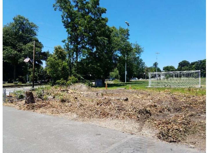
Photo depicts the tree cutting and clearing adjacent to the Woodward School soccer field on 6/25/28.
