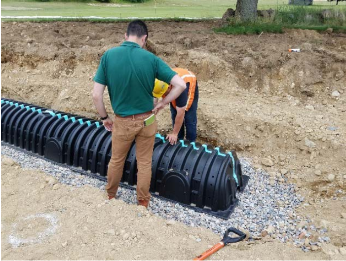
Photo depicts James Downing inspection of the septic field and septic chambers on 6/27/18.
