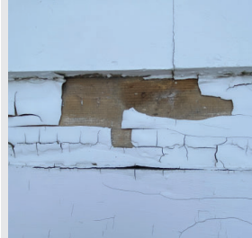
Image 18: Exterior Siding: Delaminating paint on clapboard. Alligatoring on clapboard below.
