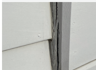
Image 22: Clapboard/Quoin Joint: Separation between quoins and clapboard in need of sealant.
