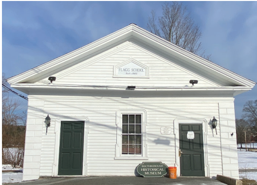
Image 15: Note the pediment featured on the main facade of the schoolhouse.
