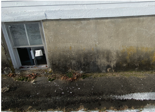
Image 29: Foundation Wall--Stains from splashing at the drip line are evident on foundation wall. Delamination at window.
