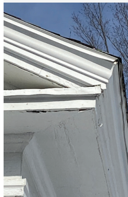
Image 21: Evidence of peeling paint at soffit.
