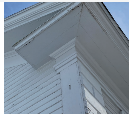
Image 13: Northwest corner: Cornerboards on north side and quoins on west side.
