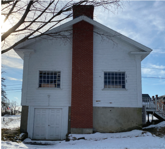
Image 16: The side cornices return to the rear facade. .
