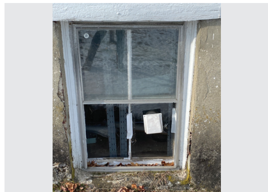
Image 27: East Elevation Basement Window--Sill is deteriorated. Storm window missing.
