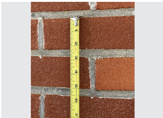
Image 11: Close up of masonry at chimney.
