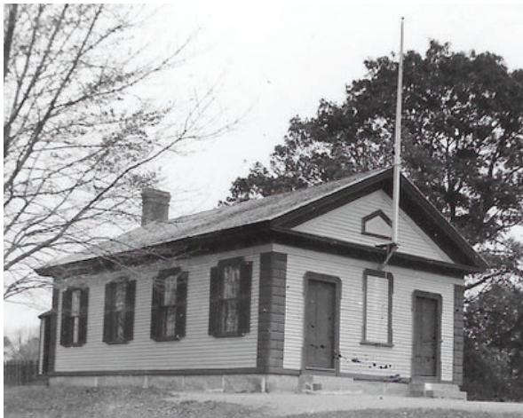
Historic Photo 1: - Probably taken in the 1880s before the building was moved to its current location showing the very dark trim paint shown in microscope photo 3A. Note the window sashes are also dark and may be the green shown in microscope photo 4. They also might be black, which was a common 19th century sash color.
