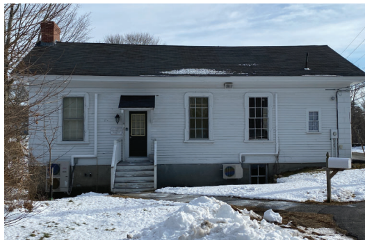
Image 8: West Elevation: The same as east elevation with plumbing vent at right and awning roof over door..
