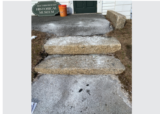
Image 32: Granite steps to main entrance: Step are of unequal rise, and pose a tripping risk. Granite block at door is tipping..
