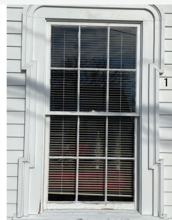
Image 14A: Example of Eared Architrave Trim: Found on the front doors and double hung windows. South facade window shown above.
