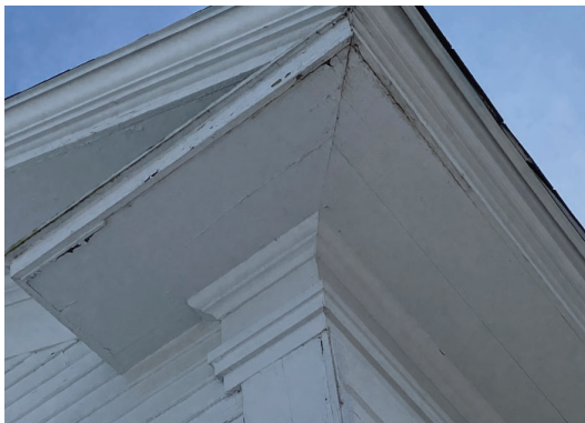
Image 17: Soffit of cornice return from west to north facade..
