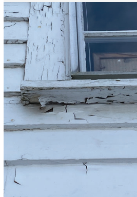
Image 19: Siding and Window Trim: Evidence of peeling paint on both..
