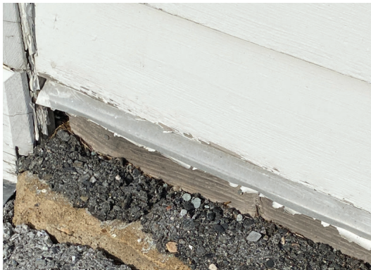
Image 30: Asphalt walkway at front facade is touching the wood clapboards.
