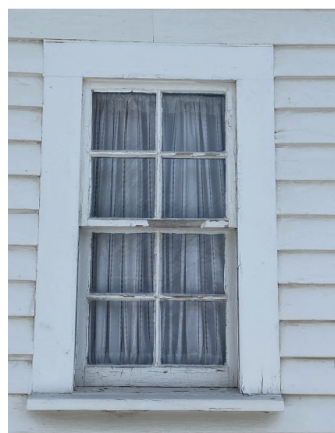
Image 14B: Example of plain trim at rear windows, small western window and basement service doors.
