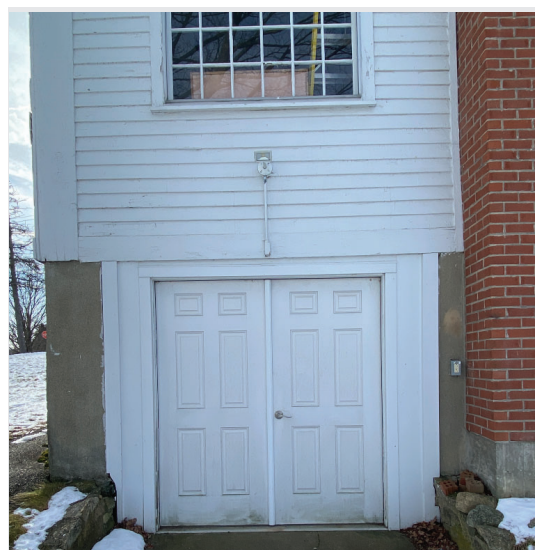
Image 28: Basement Service doors.
