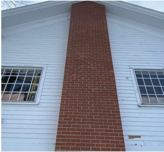
Image 9: Brick chimney on North facade
