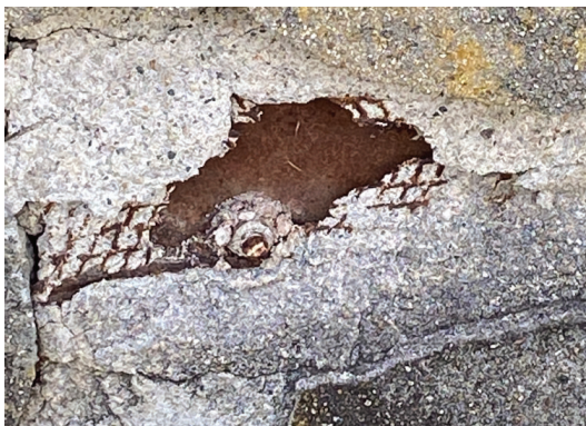
Image 31: Delamination of parging over brick foundation: Deteriorating wire mesh is visible.
