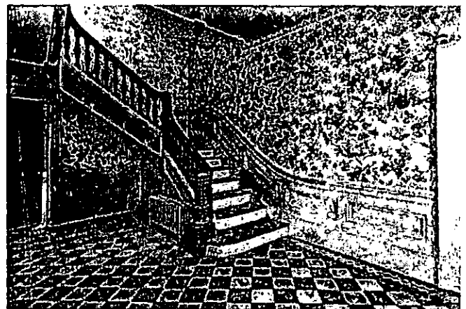
Front hall, stair
