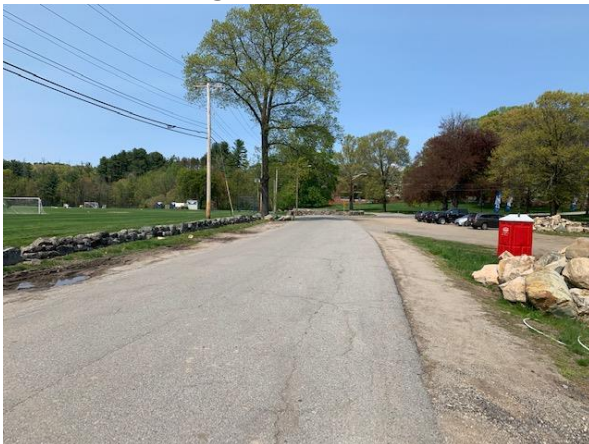
Street facing north to Marlboro Road
