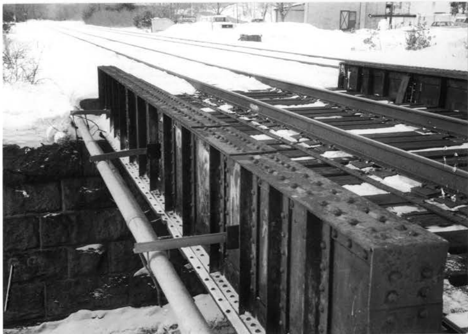
Rt. 85 Bridge under MBTA - south side plate girder.
