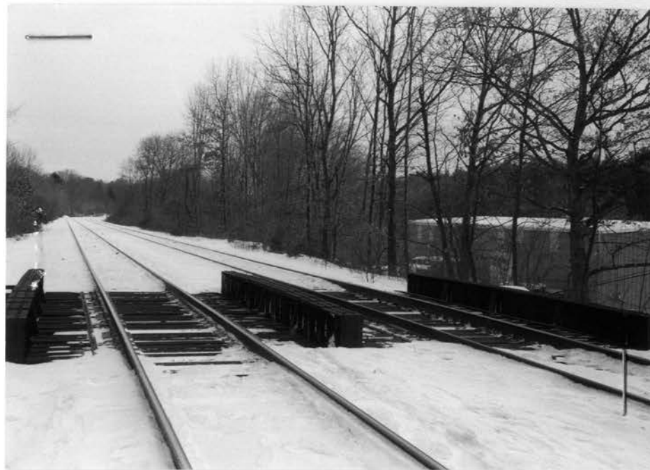
Rt. 85 Bridge under MBTA.
