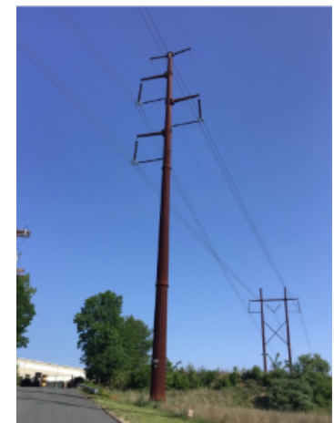
Example of a weathered Steel structure
