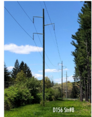
Typical D-156 wood pole structure
