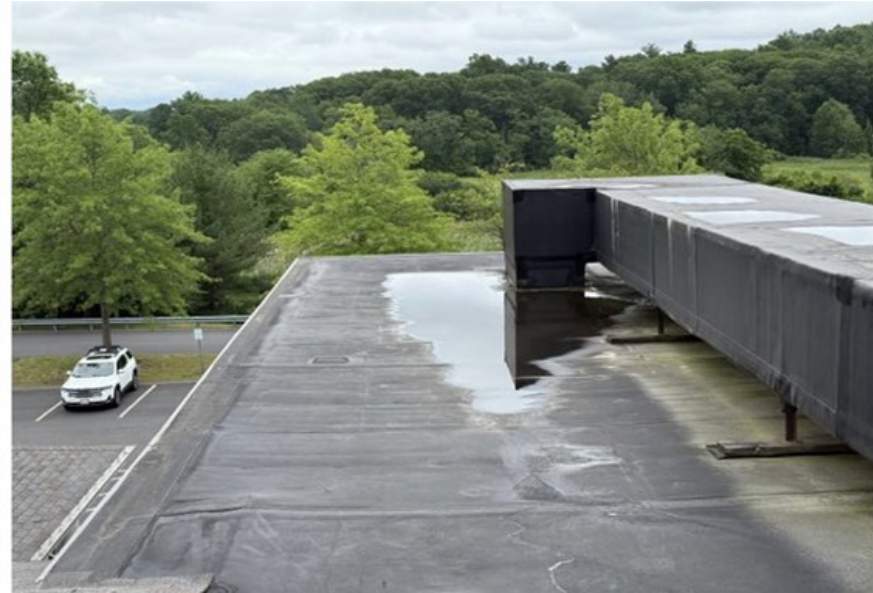
Drainage away from HVAC equipment
