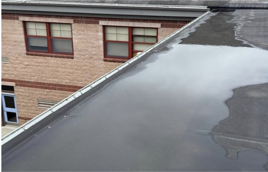
Structure for proper gutters
